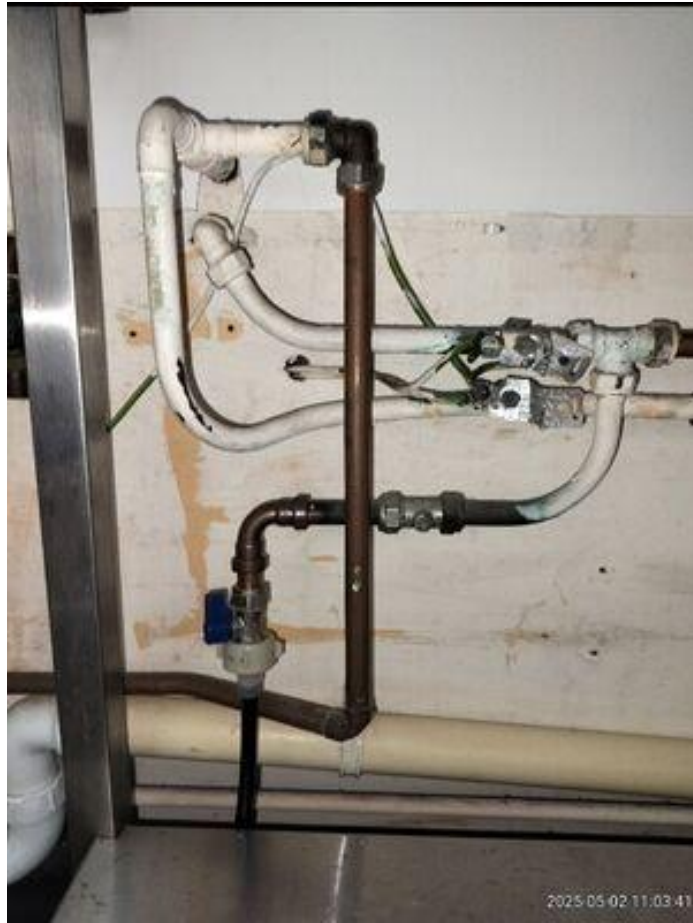
Spur to dishwasher currently open creating a dead leg
