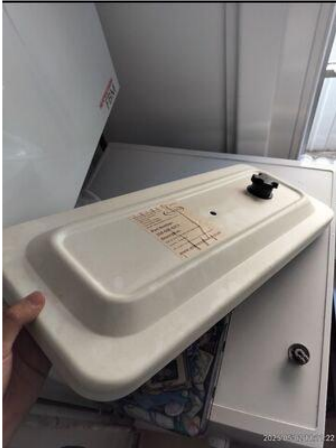
CWH 1 - External - Lid fit with a screened breather
